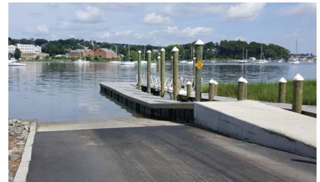
Accessible water access example.
